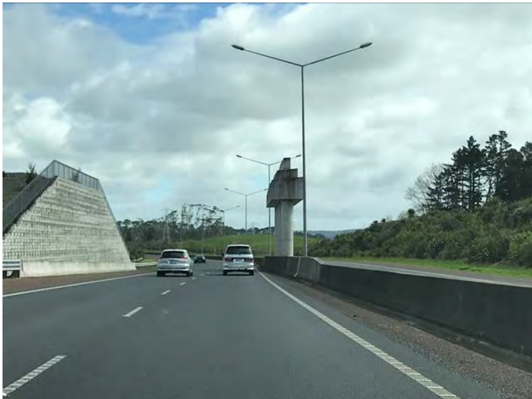
Figure 3: Pillars located on State Highway 16 to support the future Northside Drive extension
