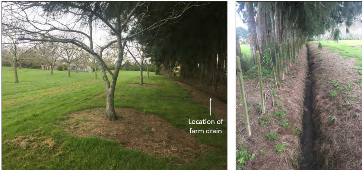
Figure 2: Photos of the farm drain located close to the boundary of the Subject Site at 12 Sinton Road
